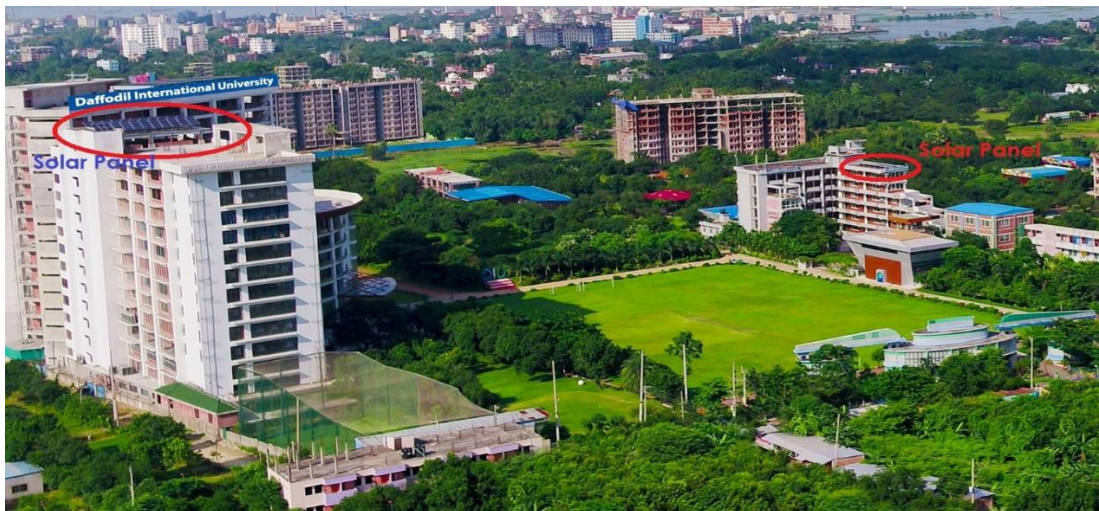
Solar panel at the roof top of Academic building 3 and 4 at Ashulia campus (Rooftop Solar Panel used for using 2000 KWH power annually)
