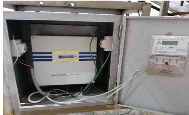
Solar panel energy grid
