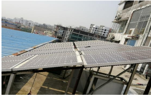
City campus rooftop Solar Panel used for using 1500 KWH power annually
