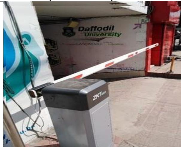
Card Touch and go system for access in the campus buildings
