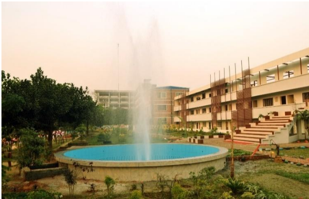
Recycled Water is used in DIU water fountain
