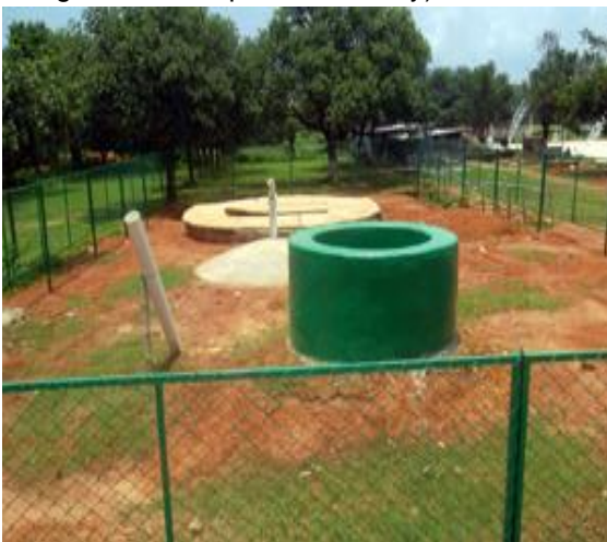
Example of Biogas plant (Daffodil International University)
