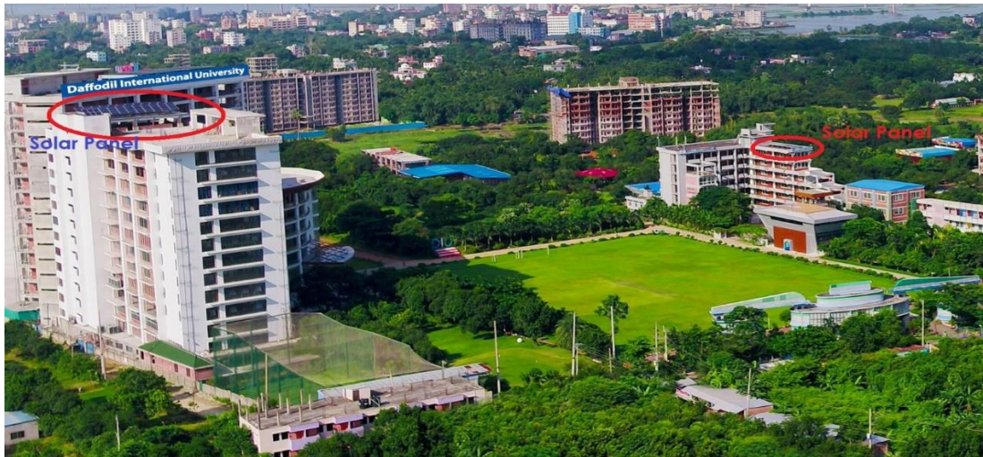
Solar panel at the roof top of Academic building 3 and 4 at Ashulia campus (Rooftop Solar Panel used for using 2000 KWH power annually)
