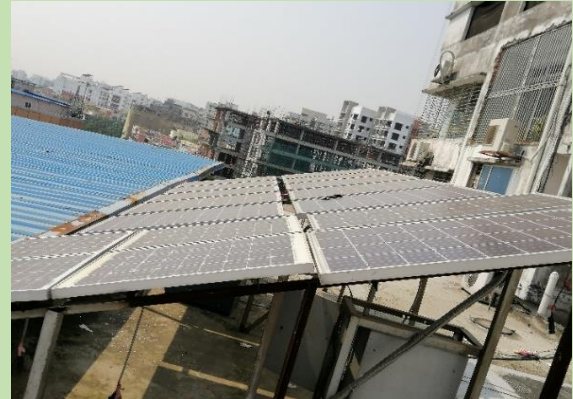
Rooftop Solar panel at main campus and city campus to reduce grid electricity consumption
