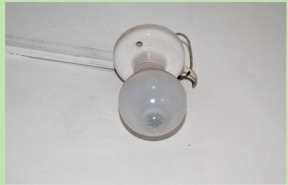
Motion Sensor based LED lights and use of reminder regarding energy efficiency
